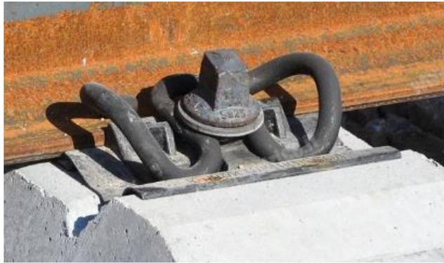
FIGURA 4 ATTACCO ELASTICO TIPO VOSSLOH
