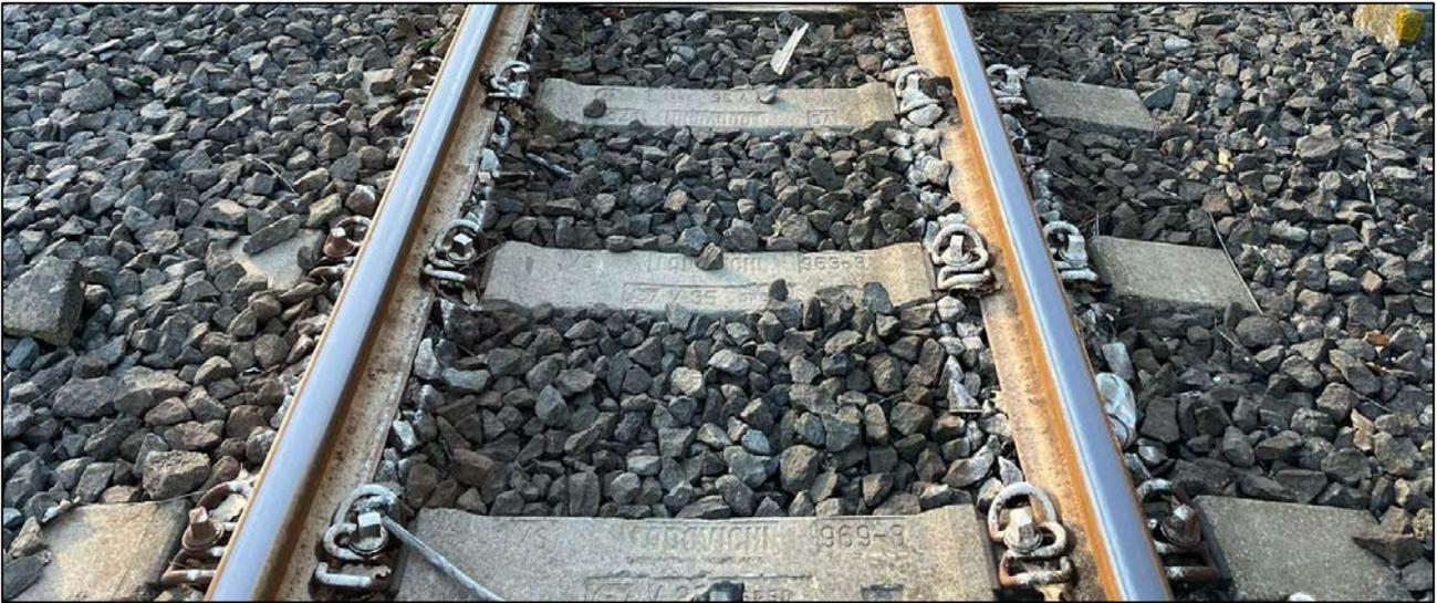
Figura 4: Traversa in c.a.p. in posa
